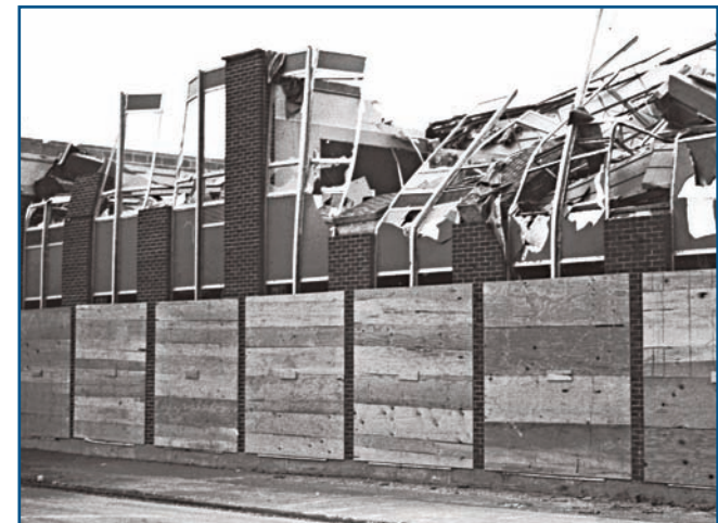
Figure 3-9 Collapsed second floor of St. Augustine Elementary School building.
