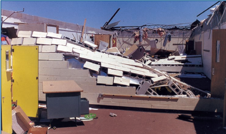
Figure 3-17 Interior and exterior unreinforced masonry walls were damaged when reinforced bond beams failed.
