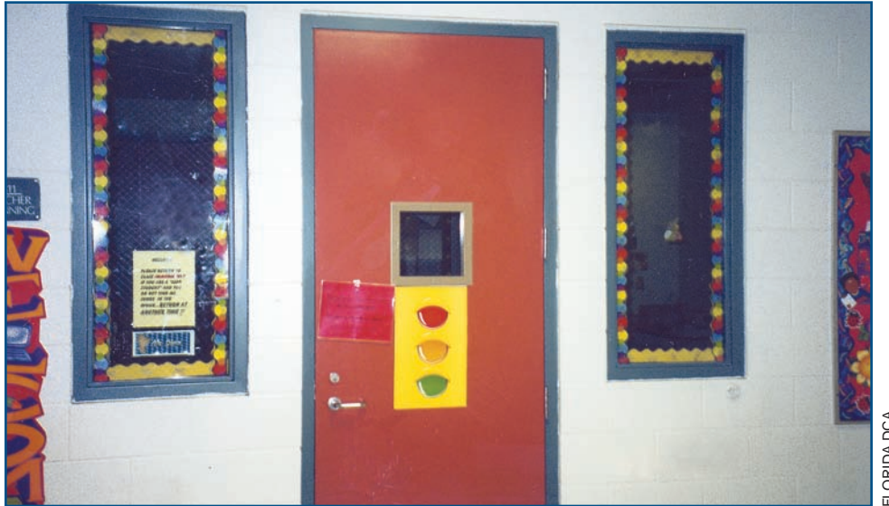
Figure 4-15 Door connecting classroom to corridor – Buildings 200, 400, 600, and 800.
