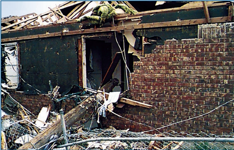
Figure 4-4 This power pole penetrated a window and extended several feet into the house after being blown 40 feet from its original location.
